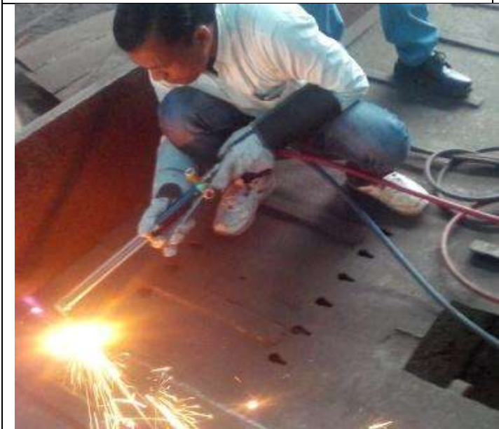
Cutting of 8 mm MS floor by CNG.
