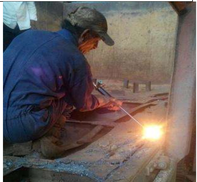
Cutting of 8 mm MS floor by CNG.
